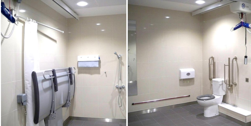
Changing Bench and Ceiling Hoist – Land-Side Changing Places
