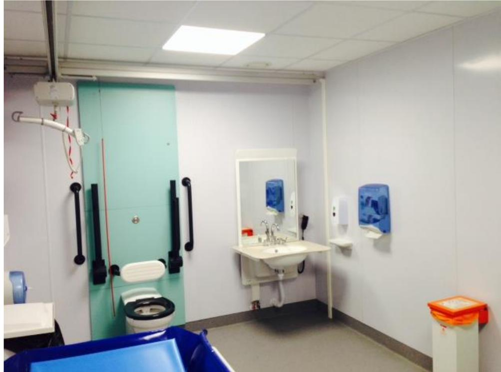
This was followed by an in-depth quotation for the Multicare mobile shower trolley and ABW6 adjustable height wash basin for additional accessibility which was accepted and manufactured to suit.
